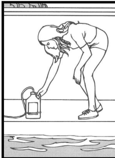
3. Place acid container on edge of pool at deep end. Carry applicator and pole to opposite side of pool.
